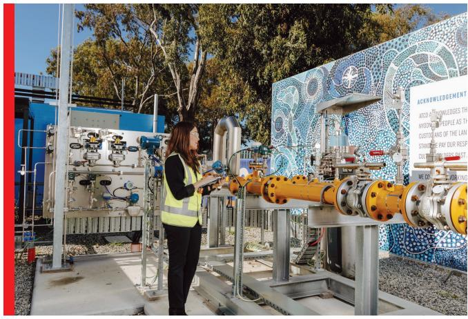
In Western Australia, ATCO has begun blending up to five per cent renewable hydrogen made at its Clean Energy Innovation Hub (CEIH) to supply 2,700 homes (picture courtesy of ATCO)
